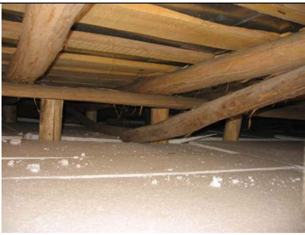
Roof insulation with Polystyrene
