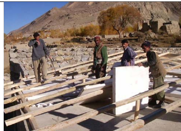
Roof insulation with Polystyrene
