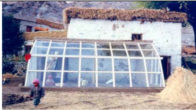
Veranda on Domestic house with thermal insulation upgrades, heating spendings reduced by 90%
