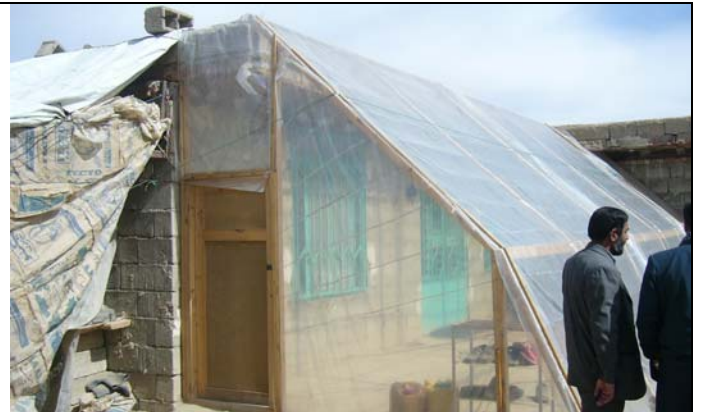
Veranda on Domestic house, heating spendings reduced by 50%
