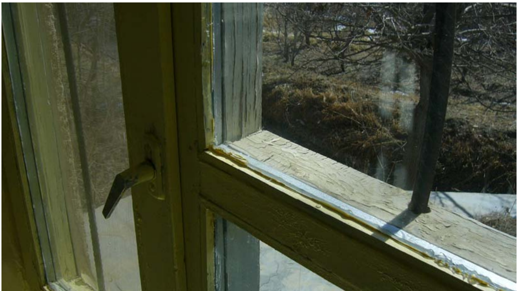
Overglazing with Silicone sealant on existing wood frame
