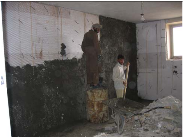
Inside insulation (renovation) with Polystyrene
