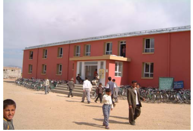
Laghmani School North face
