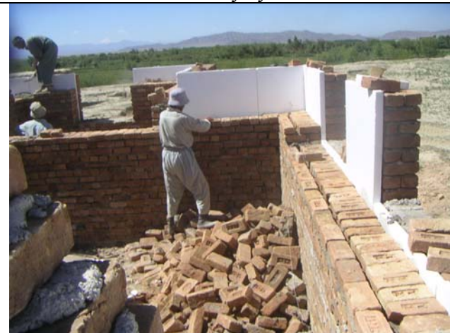
Insulated double wall with Polystyrene
